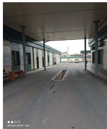
Garage service pit
