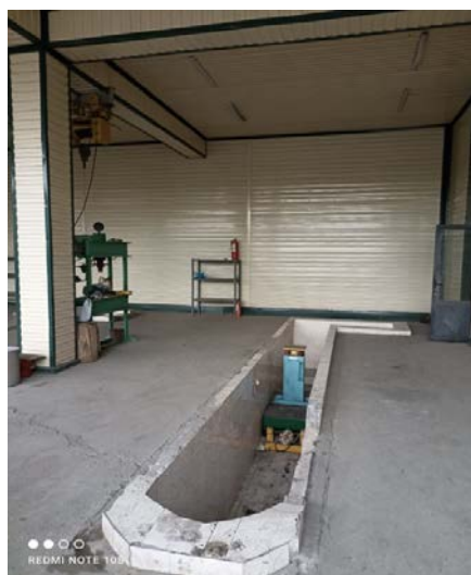
Area of minor repairs
