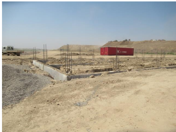
Pic. 4 Earthworks in the administrative area (28.07.2023)
