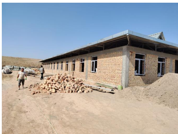
Pic. 9 Construction works on management area facilities (01.11.2023)
