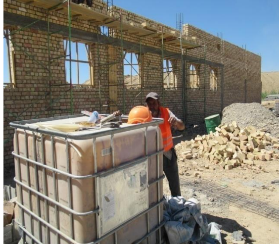
Pic. 6 Brickwork of the walls of the administrative building (14.08.2023)
