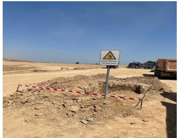
Pic. 2: Installed warning sign and protective tape
