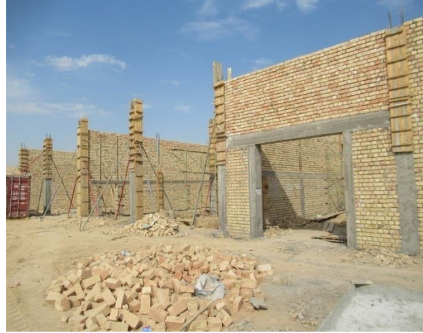
Pic. 4 Construction of administrative building (27.09.2023)
