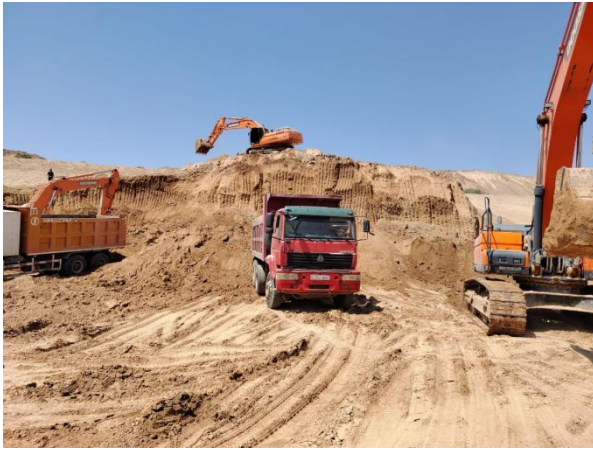
Pic. 5 Earth works (27.08.2023)
