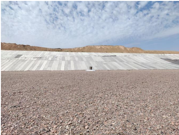
Pic. 7 liner system installation (15.09.2023)
