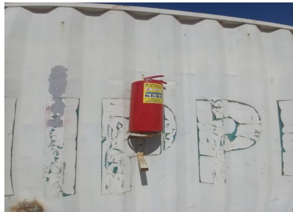
Pic. 4 Faulty fire extinguisher replaced with a new copy
