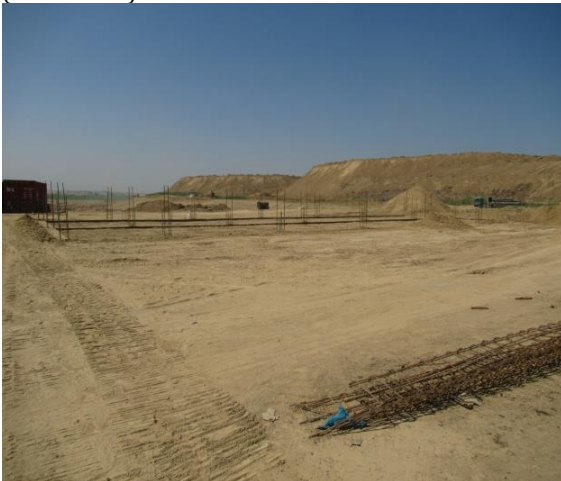
Pic. 9 Filling foundation of administrative building (09.06.2023)
