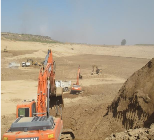
Pic. 5 Earthworks in the lower part of the facility (23.07.2023)
