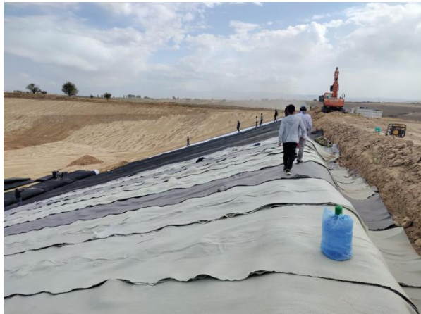
Pic. 8 Liner system installation works (02.10.2023)
