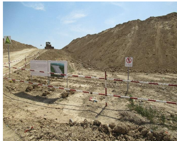
Pic. 2 Installed barriers, road signs and warning signs around the Site (06.06.2023)
