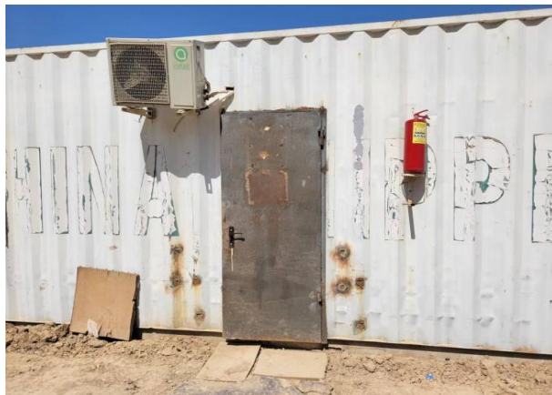
Pic. 3 Fixed trailer door for temporary rest of staff
