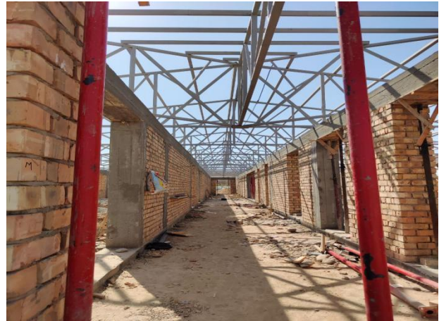
Pic. 6 Construction of administrative building (23.08.2023)
